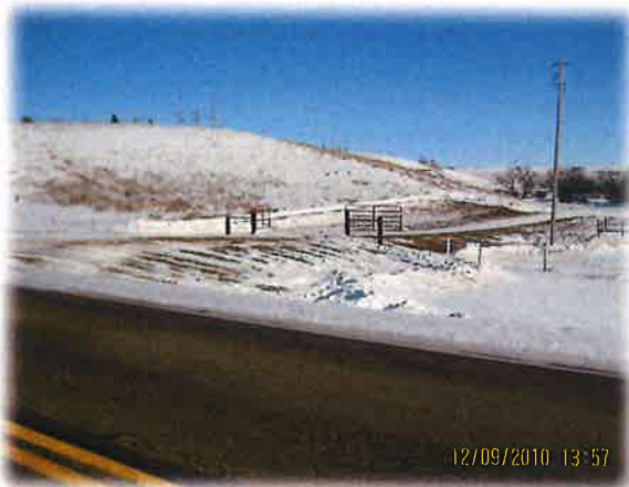
Example of proper snow removal around driveway, snow is pushed away from roadway.
