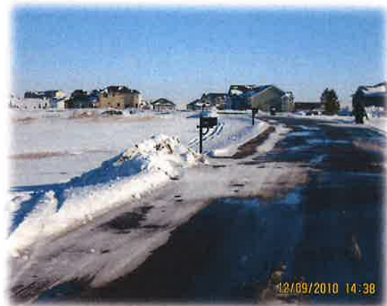
Example of improper snow removal, snow is piled along roadway.
